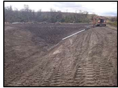
Figure 13. Chuckhole site under construction.
