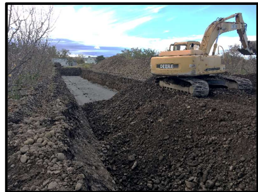
Figure 20. Locust Road site under construction.
