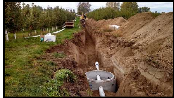
Figure 19. LeFore site under construction.
