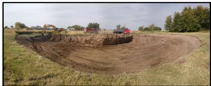
Figure 21. Mud Creek site during construction.
