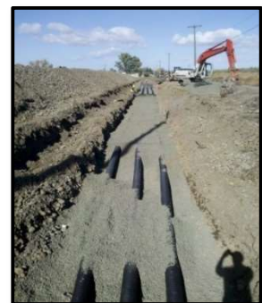
Figure 24. Trumbull site under construction in October 2012.
