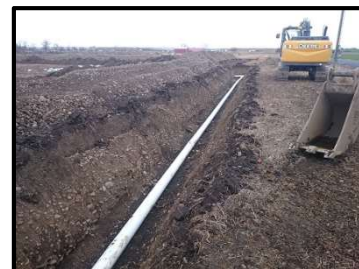
Figure 15. Fruitvale site under construction.
