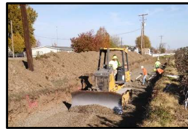
Figure 14. East Trolley Lane site under construction.
