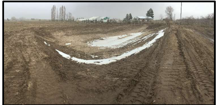
Figure 23. Triangle Road site under construction in fall 2016.
