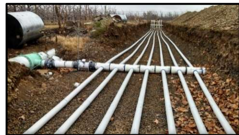
Figure 12. Barrett site under construction.
