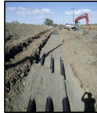
Figure 20 - Trumbull site under construction in October 2012.
