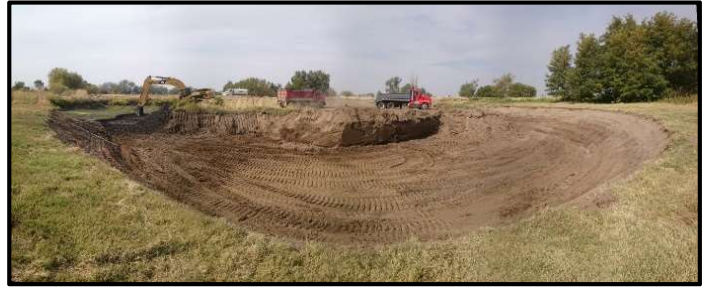
Figure 17 - Photograph of Mud Creek site during construction.
