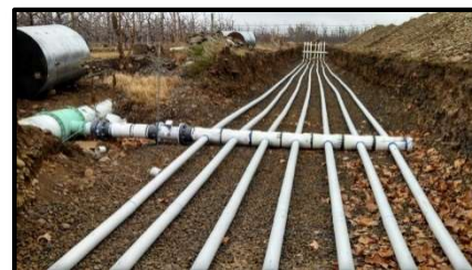
Figure 11 - Barrett site under construction.
