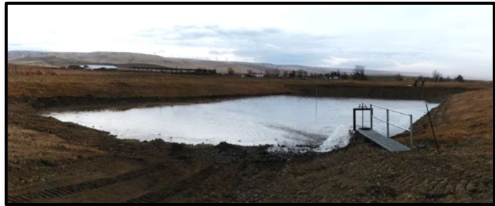
Figure 18 - NW Umapine site during WY2014 recharge season.
