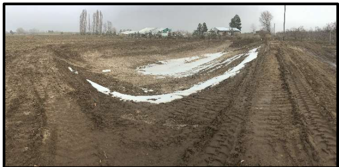
Figure 19 - Triangle Road site under construction in fall 2016.
