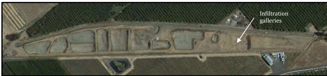
Figure 15 - Aerial photo of the Johnson site in 2013 showing 10 basins and location of infiltration galleries.
