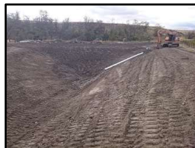
Figure 12 - Chuckhole site under construction.
