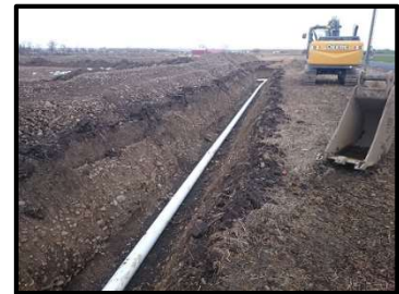
Figure 13 - Fruitvale site under construction.
