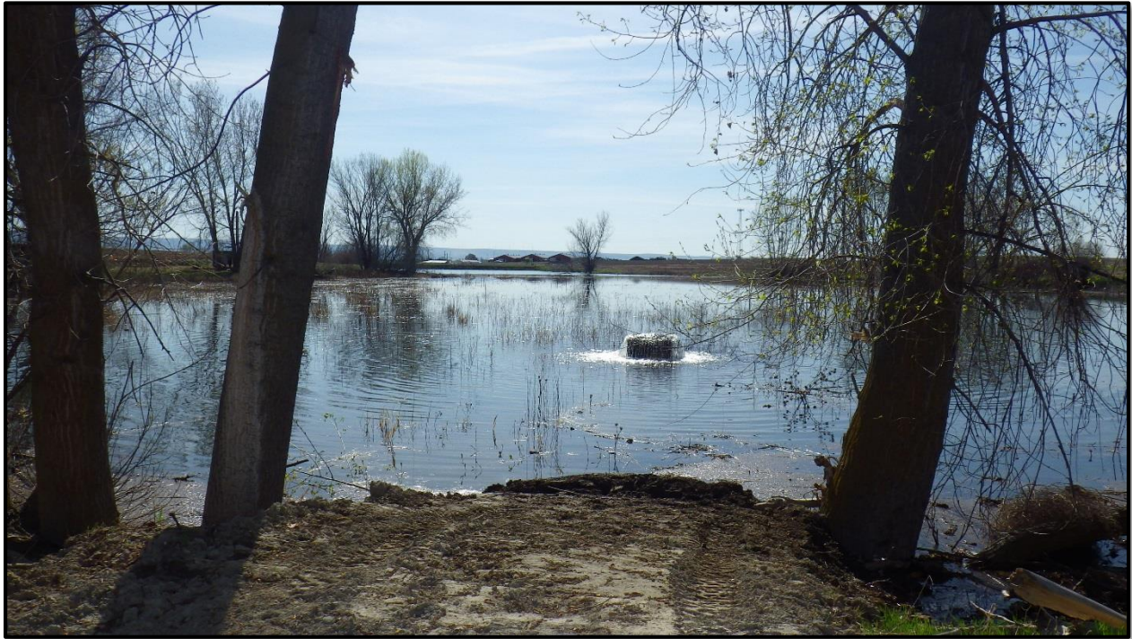
Figure 16 - Stiller Pond Aquifer Recharge site during operations.
