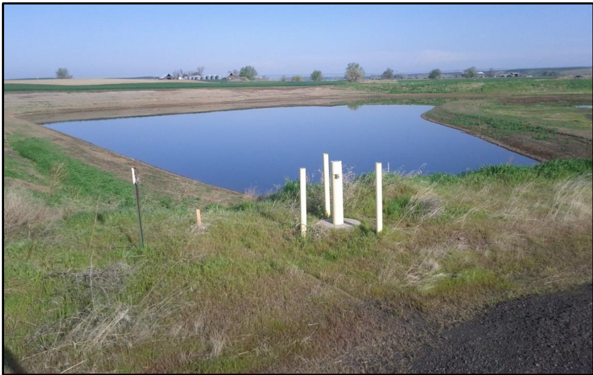
Figure 14 - Photo of the Locher Road aquifer recharge site during operations.
