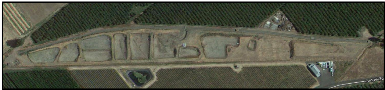
Figure 14 - Aerial photo of the Johnson site from 2013 showing the current configuration of the site with 10 spreading basins and 3 active infiltration galleries (between the spreading basins and the pile of fill material).
