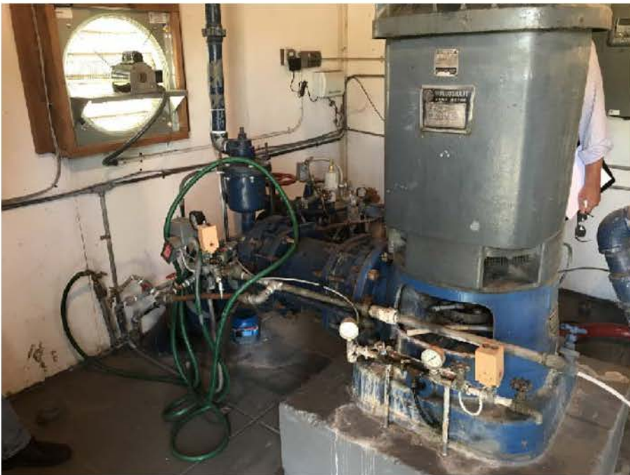
Well #1 inside looking west
