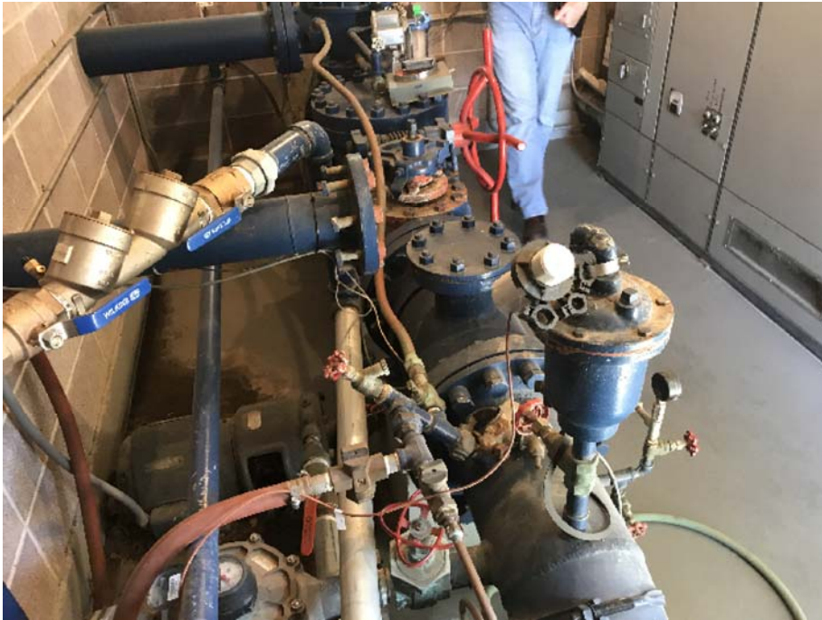
Well #8 inside north end
