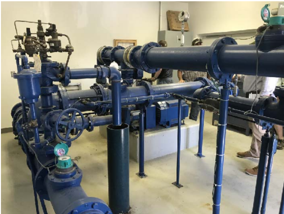
Well #9 inside looking east
