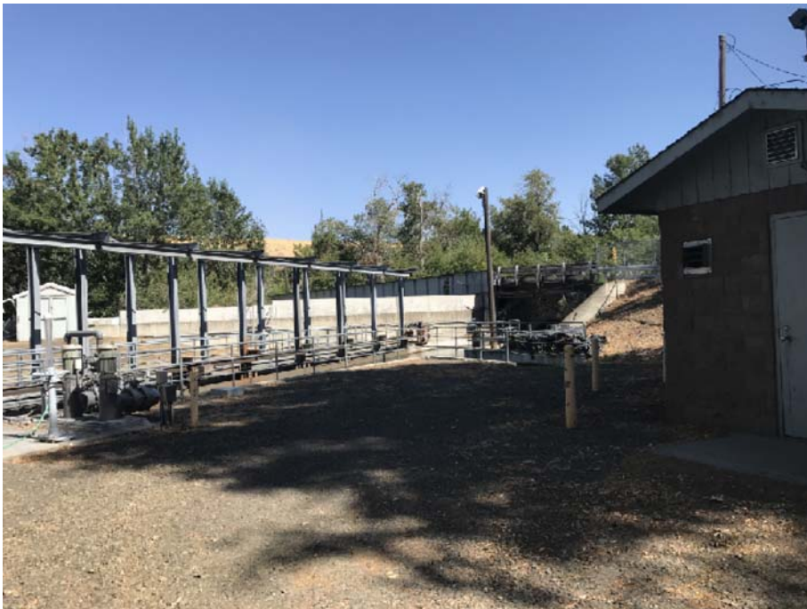
Diversion at Little Walla Walla River
