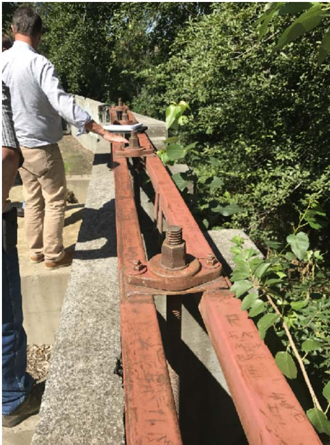
Diversion at Little Walla Walla River
