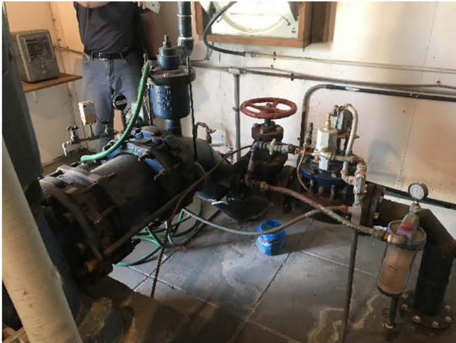
Well #1 inside looking east
