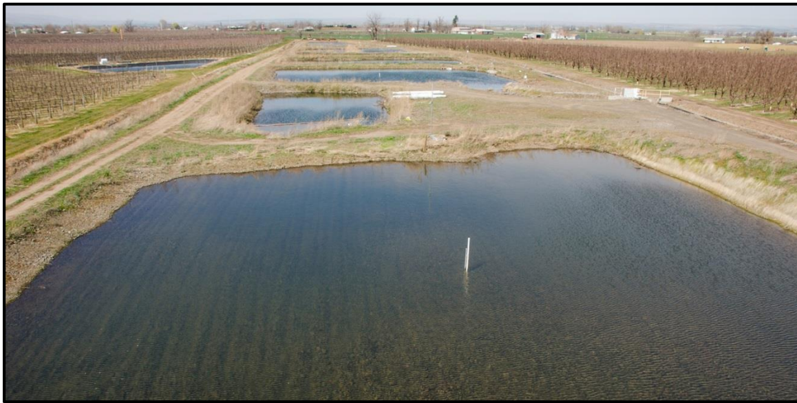
Figure 14 - Photograph of the Johnson AR site showing the infiltration basins at the site. Photo is looking northwest from the most up-gradient basin.
