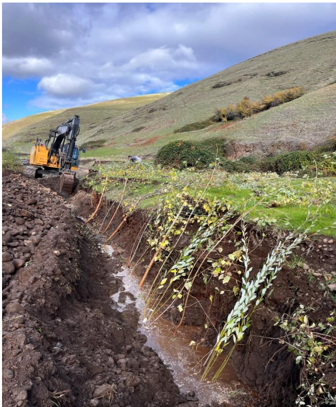
Figure 14. Willow trenching is a part of design specs to be performed cooperatively with WWBWC.
